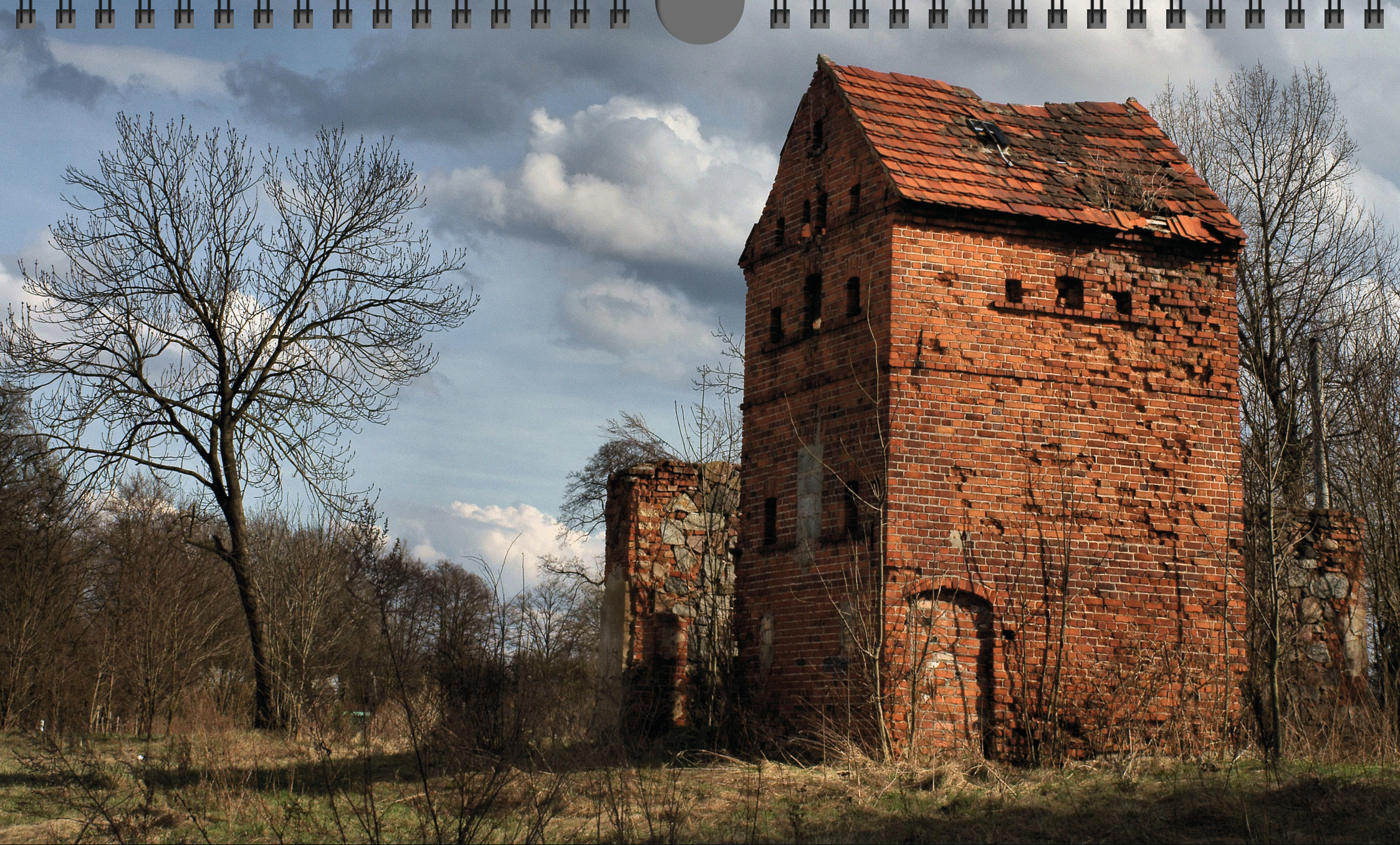
Former vodka distillery in Komorniki, Polkowice, Poland, by Zetem
