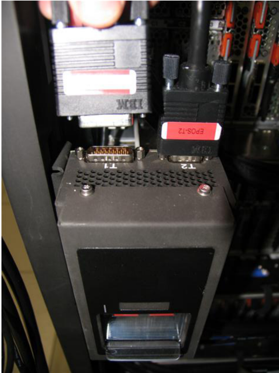
Figure 13 UEPO Cable Removal
