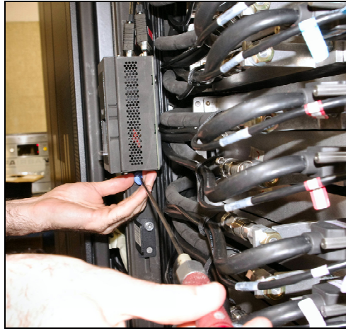
Figure 14 Removal of UEPO Panel from Frame
