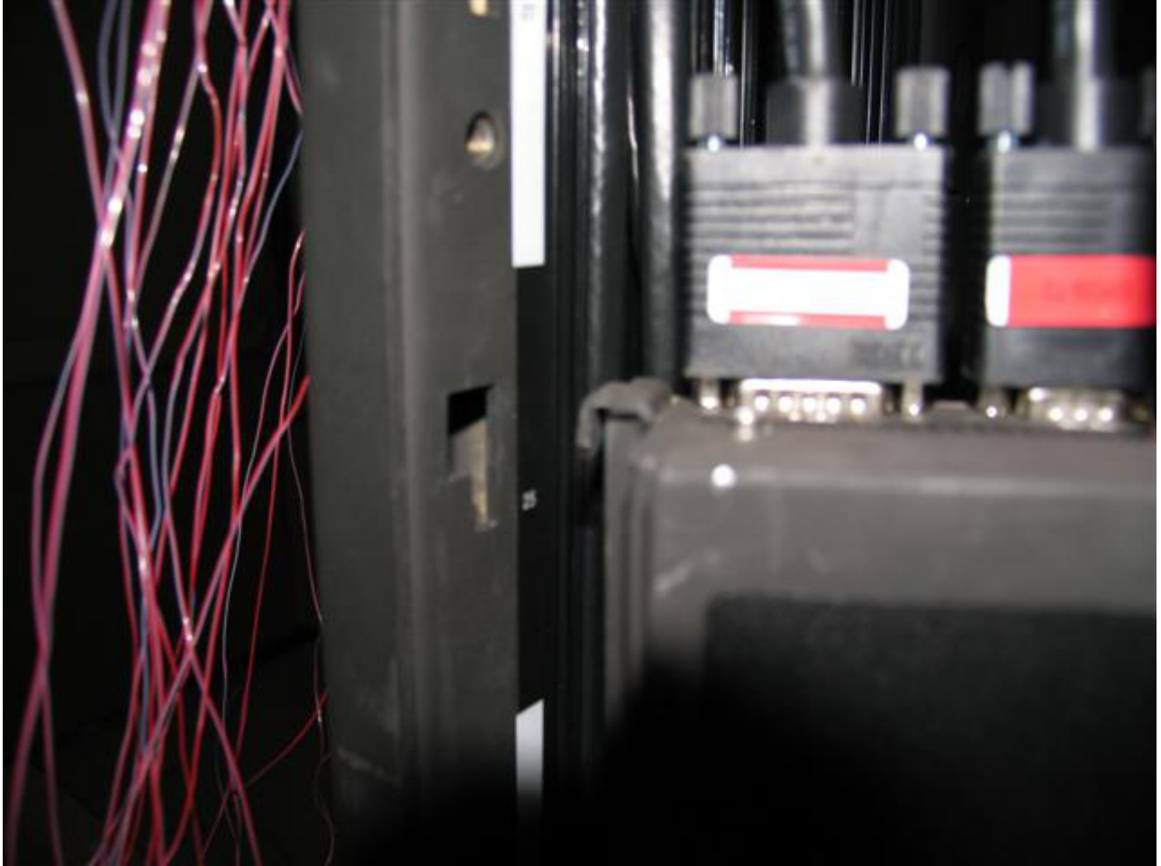
Figure 15 UEPO Panel Hook Tab & Frame Member Slot
