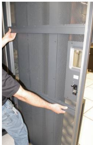
Figure 10 Removal of Front Door
