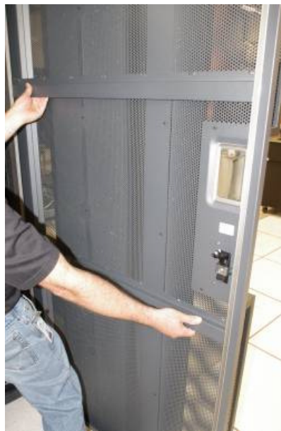
Figure 13 Removal of Front Door
