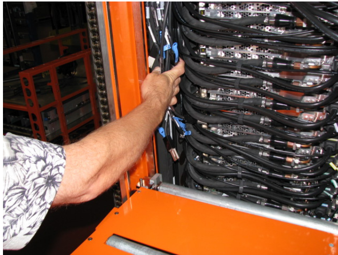
Figure 37 Relocate the DCCA cables
