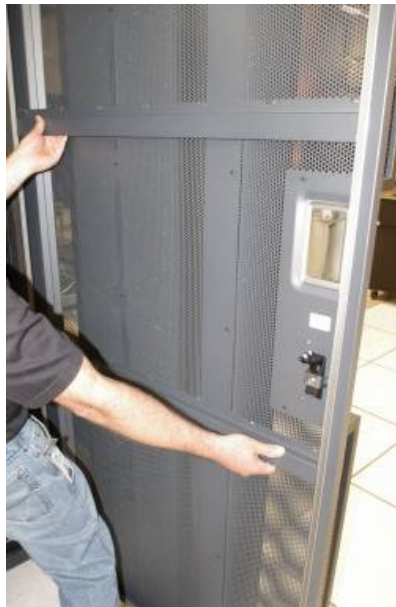
Figure 12 Removal of Front Door
