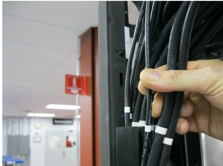
Figure 13 Communications Cable Removal
