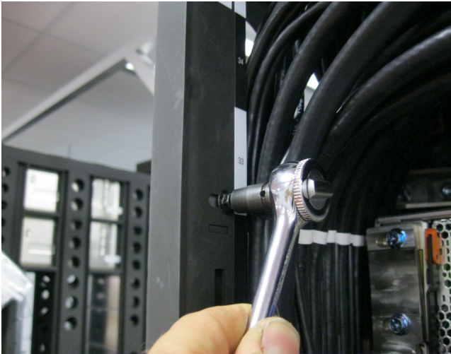
Figure 13 Raceway Retention Screw
