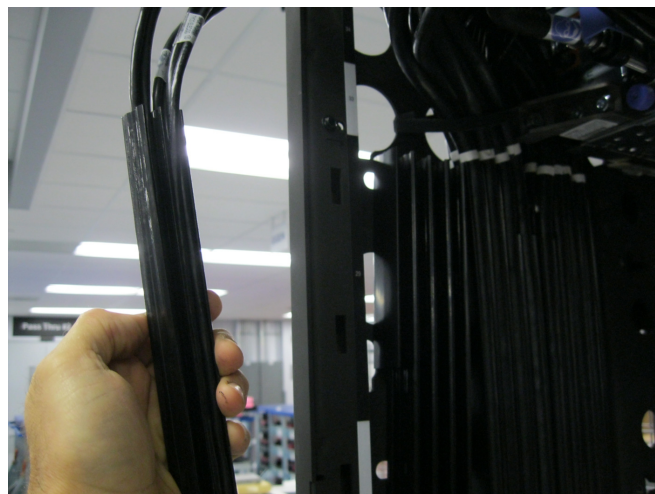
Figure 14 UPIC Raceway Removal
