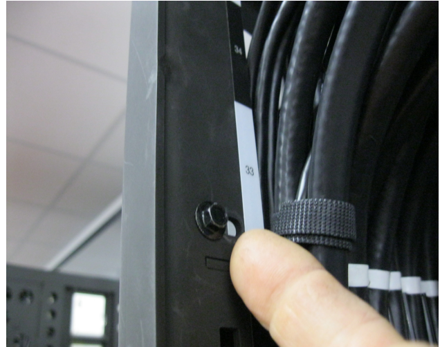
Figure 13 Raceway Retention Screw
