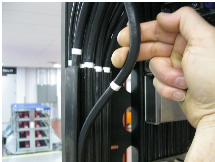
Figure 16 DCCA Power Cable Removal
