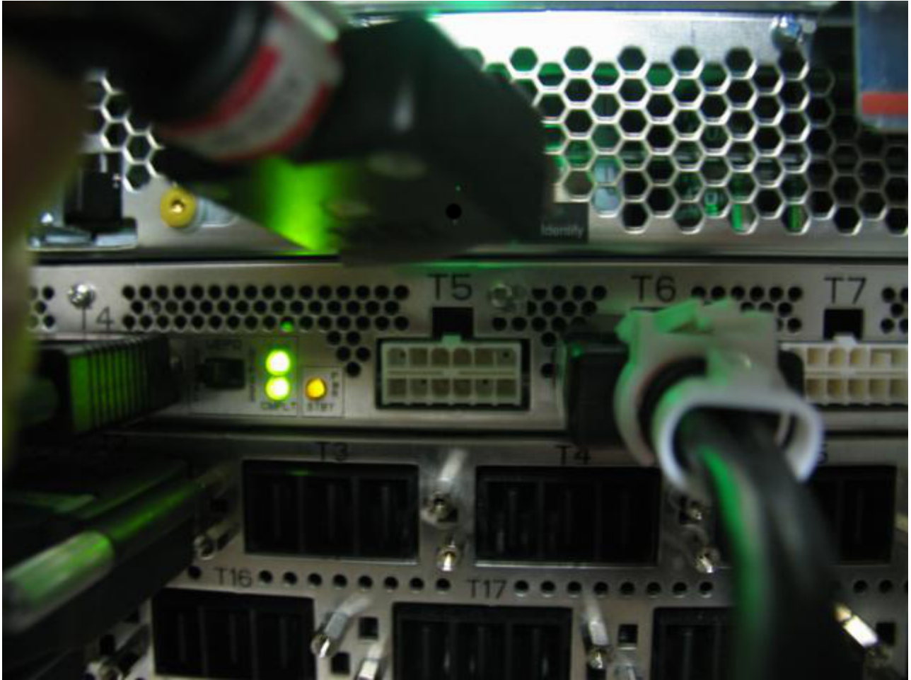
Figure 9 Removal of Cross-Power Cable from BPCH T5
