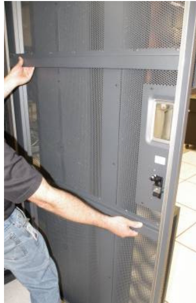
Figure 10 Removal of Front Door
