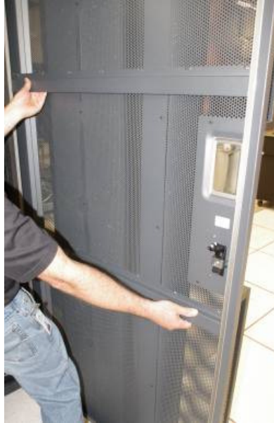
Figure 10 Removal of Front Door
