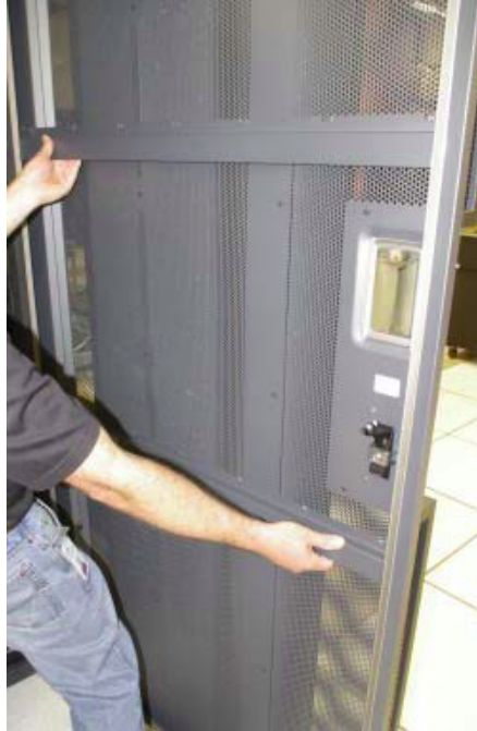
Figure 6 Front Door Removal
