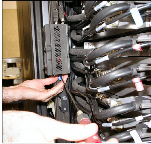
Figure 10 Removal of UEPO Panel from Frame
