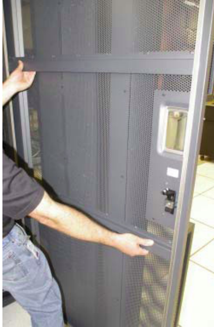
Figure 58 Front Door Install
