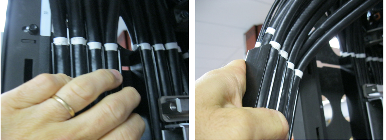
Figure 20 HPIC Raceway Removal
