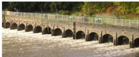
Abbey Mills Pumping Station
