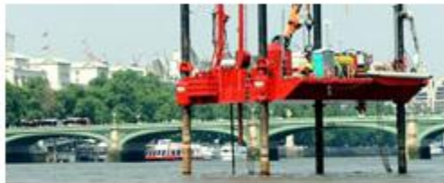
Exploratory works for the Thames Tunnel
