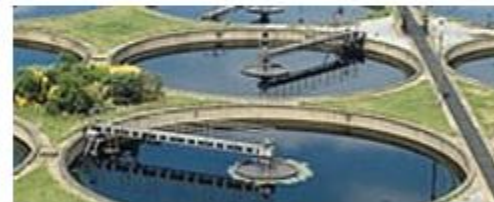
Mogden Sewage Treatment Works
