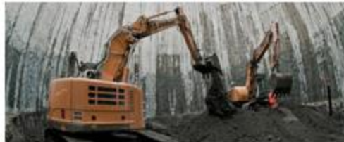
Lee Tunnel shaft under construction
