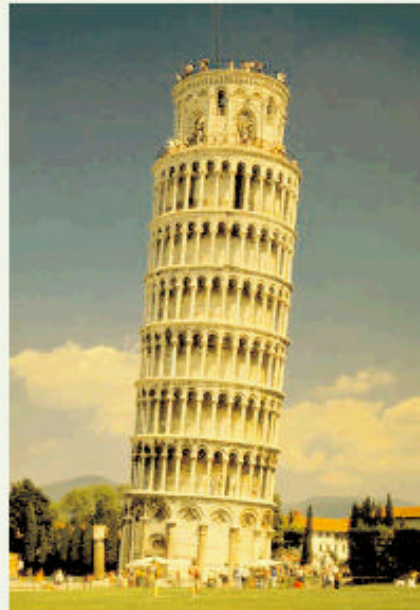
Nice facade. Bad infrastructure.
