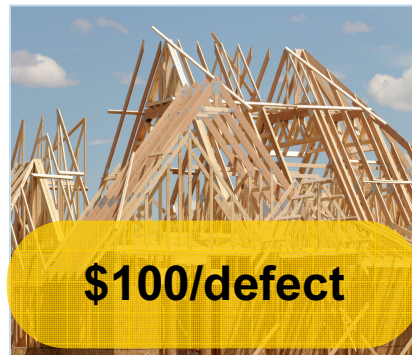
During the build phase
