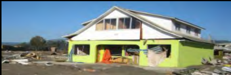
House in Pelluhue with solid first floor resisted the tsunami
