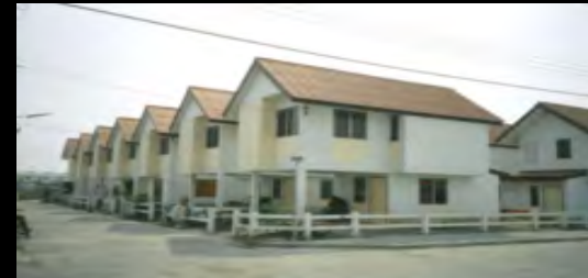
Houses with a tsunami resilient design constructed in Indonesia
