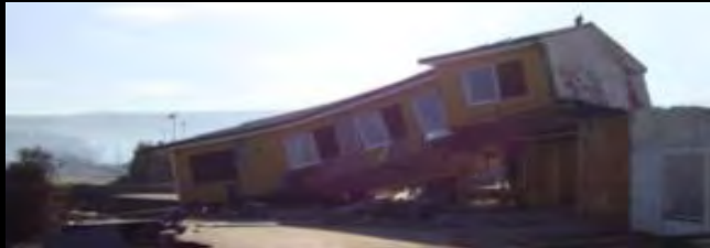
No resistant tsunami houses in Dichato
