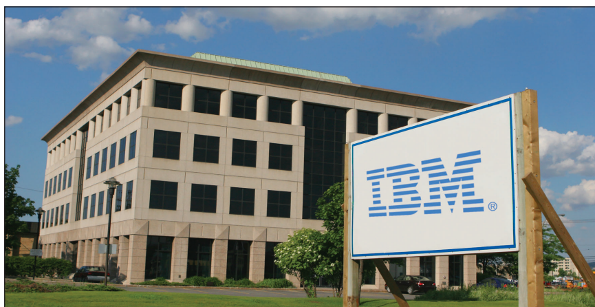
A Property Performance Management solution is providing IBM with an holistic view of all assets within its property portfolio
