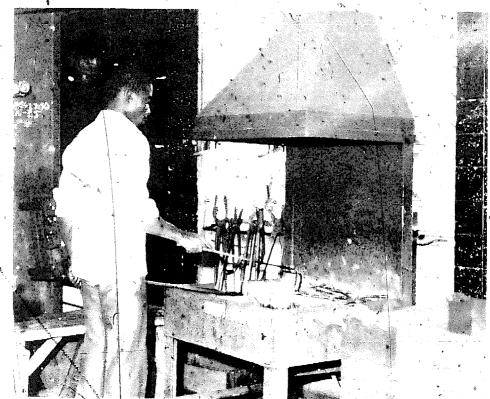
horging coach holts; bolt heads being heated in locally made blacksmiths hearth at the TCO Workshop 1974.
