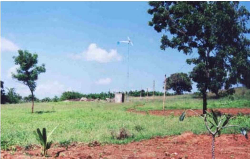
Photo 9: A wind generator on an open site. The tower should be as tall as possible, and well above the tree tops. (Simon Dunnett, Sri Lanka)
