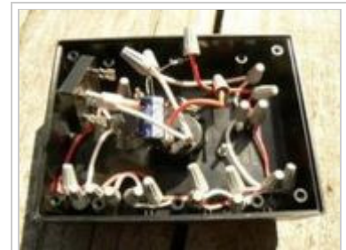
Inside LED meter box
