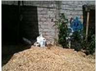
Fig. 1: Tank area before hole was dug
