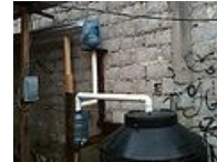
Fig. 4d: First flush system all set up
