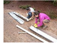
Fig. 4e: Gabby and Bri prepping gutters for wiring
