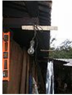
Fig. 2f: Wood supports
