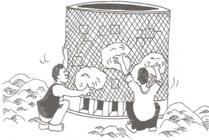
Figure 4.19 Plastering the kiln wall
