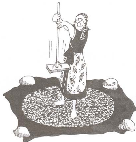
Figure 4.4 Levelling the foundation
