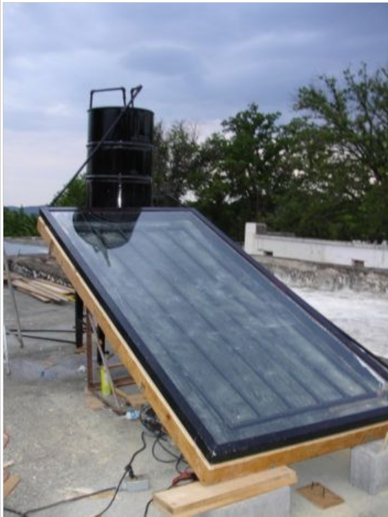
Closed Loop Passive system in Parras de la Fuente, Coahuila Mexico
