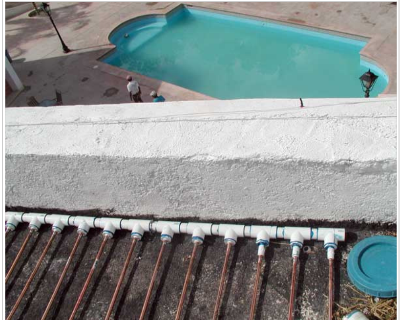
Solar hot water system for a hotel in Parras de la Fuente, Mexico
