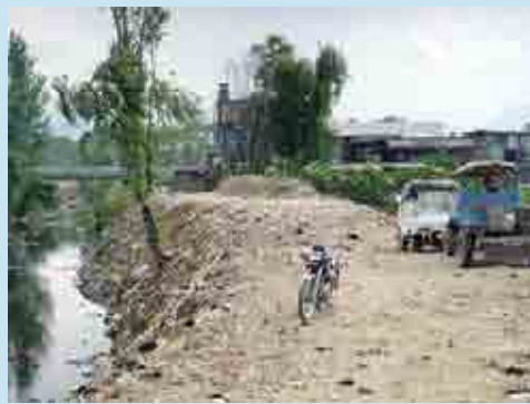
Filling with cover material (soil)
