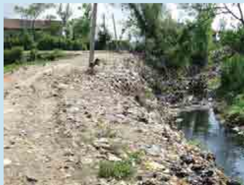
Road on old dumped waste
