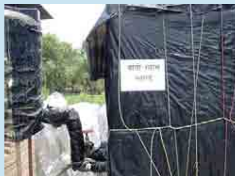
Biogas plant at WEPCO
