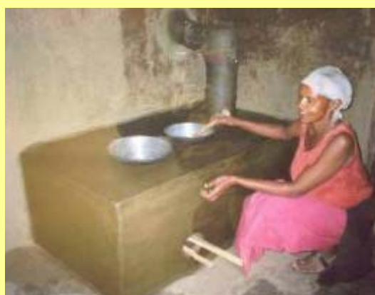
In-built rocket Lorena – double pot, chimney, mud/bricks. Photo: GTZ
