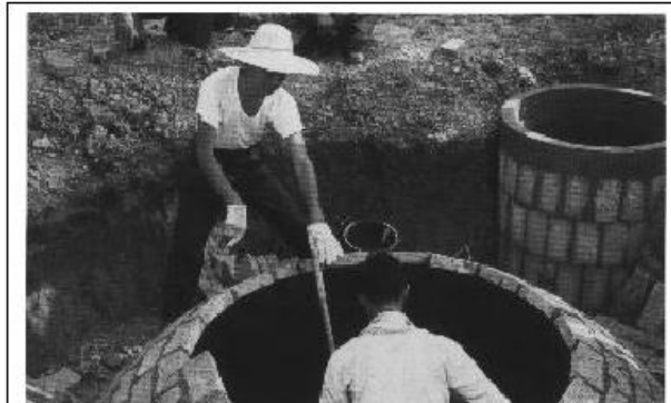
Figure 6: Installation of a Shanghai fixed-dome system near Shanghai, PR China
