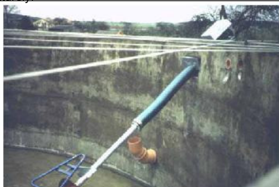
Figure 32: Mixing device in an agricultural digester under construction
