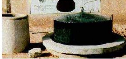
Figure 7: Floating-drum plant in Mauretania Photo: gtz/GATE
