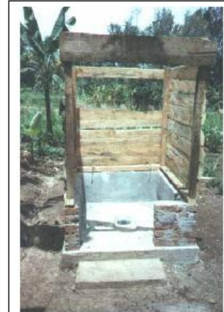
Figure 16: Toilet (under construction), directly connected to the plant Photo: Kellner (TBW)
