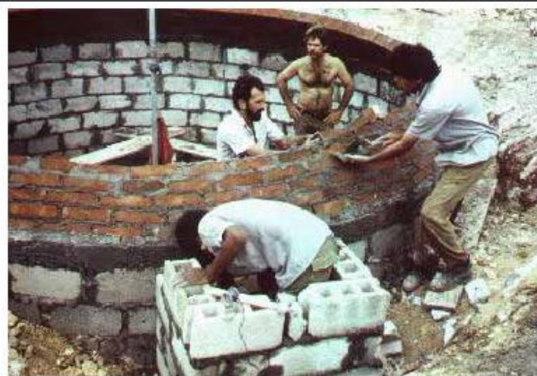
Figure 17: Construction of the dome for a 30 m 3 digester in Cuba
