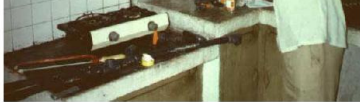
Figure 26: Final touches on a piping system with PVC pipes
