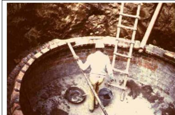
Figure 21: Construction of the weak/strong ring of a 16 m 3 , Tanzania
