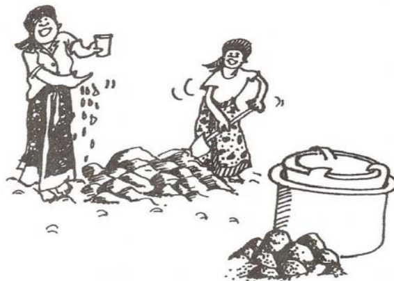
Fig. 7.2 Mixing murrum with water
