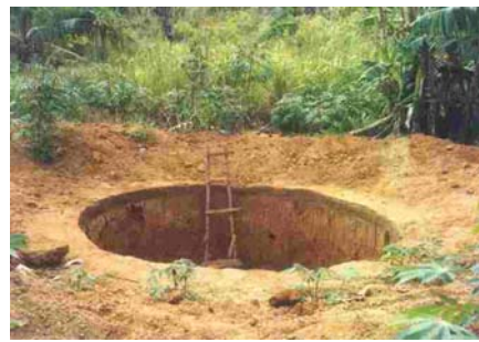
Figure 3: Pit for the tank construction
