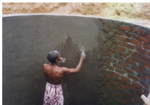
Figure 12: Plastering the tank
