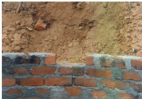
Figure 10: Outlet of the tank before plastering
