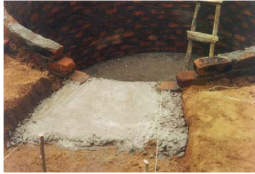
Figure 7: Concrete base for the inlet construction
