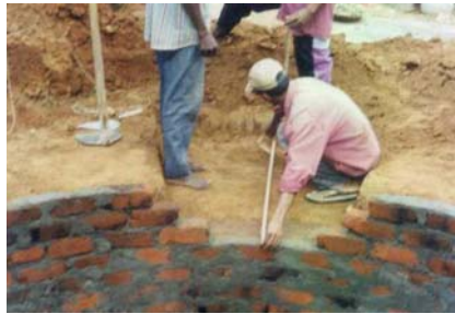
Figure 6: Measurement taken for the inlet construction
