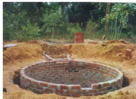
Figure 11: Completed tank before plastering
