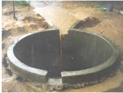
Figure 13: Run off rain water collection to the tank
