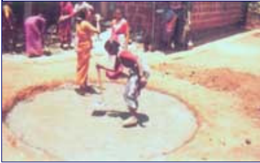
Lay the foundation
