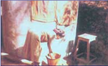
Cure the structure by draping wet hessian sacks
