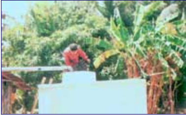
Filling the filter with filter media
