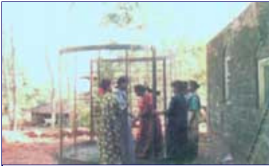
Erect the mould skeleton
