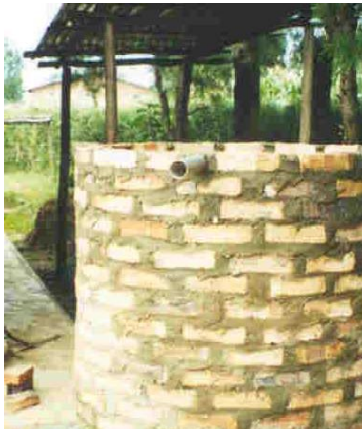
Figure 4 Full height of the brickwork clearly showing the position of the overflow
