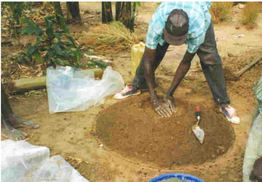
Figure 1 Mould for brick jar cement cover
