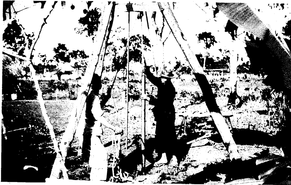
Fig. 19 Bailing well with 6 cm diameter bailer
