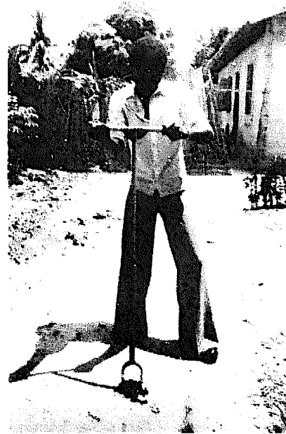
Fig. 44. Test drilling is normally started with a combination auger of 100 mm diameter.
