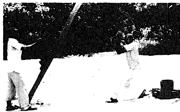
Fig. 71. Bailing in coarse sand or gravel. The winch operator should exactly follow the instructions of the person who is bailing.
