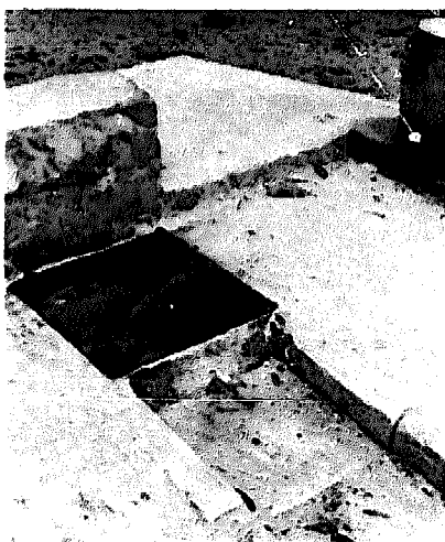
Fig. 137. During repairs the well must be covered.
