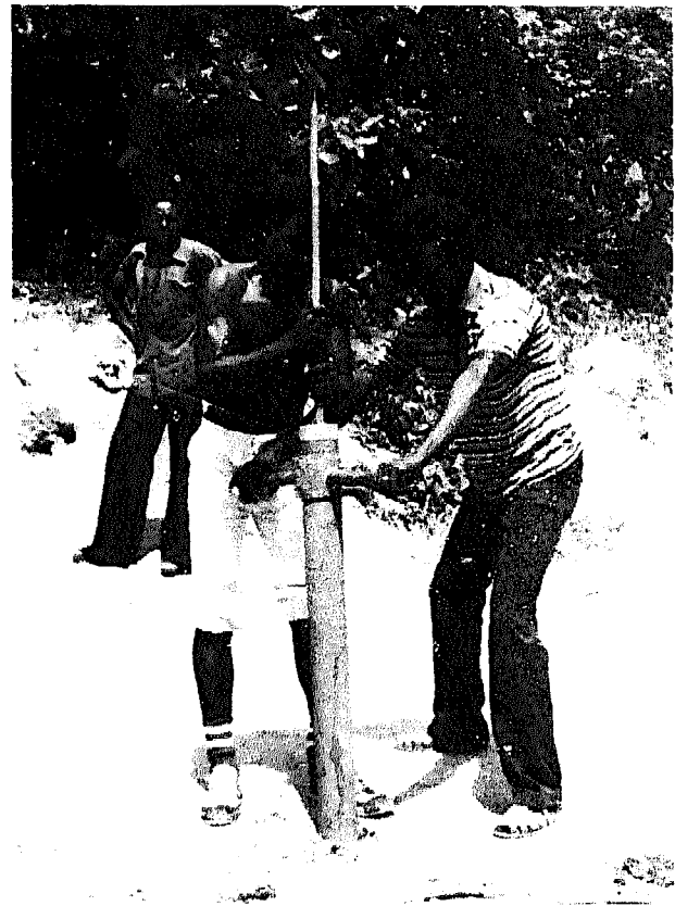
Fig. 48. The casing has to be lowered while bailing and is rotated clockwise.
