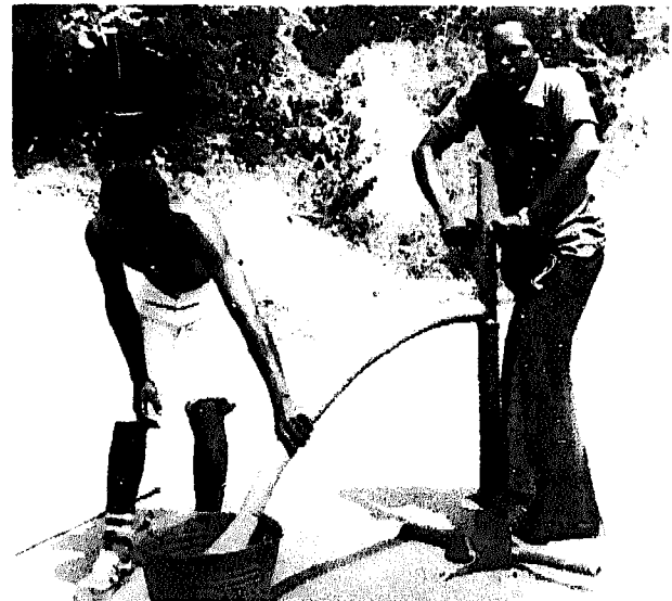
Fig. 49. Survey test pumping. In order for the casing not to be damaged by the foot plate of the pump, a steel head is screwed on top of the casing.
