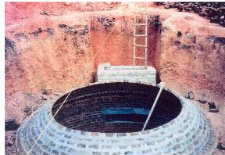
Fig. 9: Biolatriner for 2x3 toilets, 200 people in Kumasi, Ghana (under constr.) front: digester, rear: influent shaft (Source: [β])
