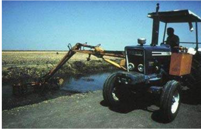
Slide J.19 Mechanical weed clearance of canals
