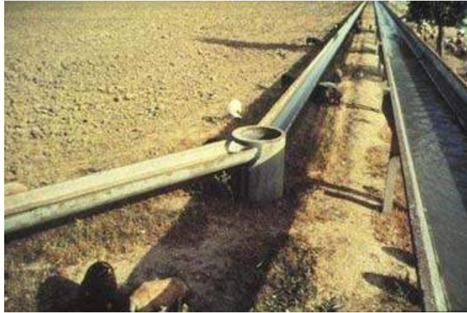
Slide F.8 Lined canal and canaletti, Morocco
