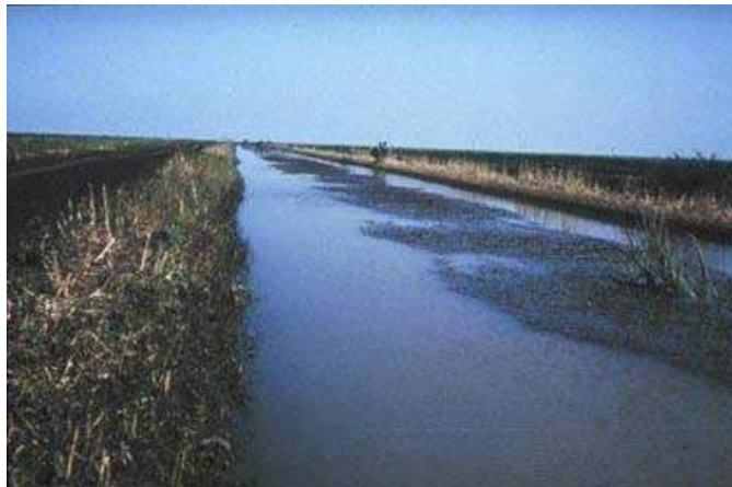
Slide F.20 Minor canal with aquatic weeds, Rahad, Sudan
