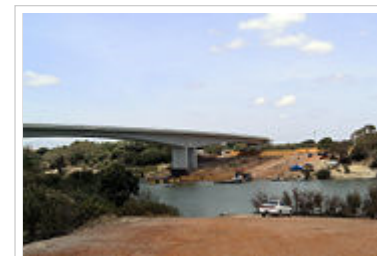
Cross-border bridge from Guyana to Brazil under construction near Lethem.
