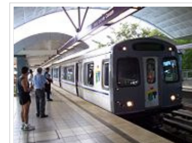
Tren Urbano at Bayamón Station
