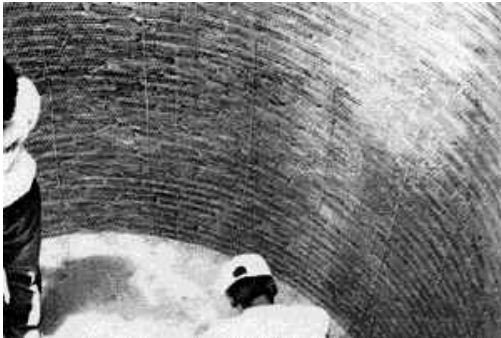
Figure 3 - inner tank wall surface showing wire mesh in place
