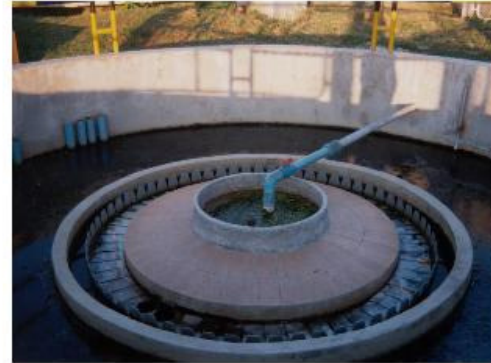
Fig. 2: Pig slaughterhouse Phitsanulok, Thailand: Influent distribution system to UASB reactor
