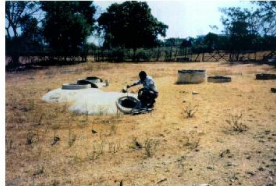
Fig. 3b: effluent point; rear left: digesters, rear right: manhole of digester
