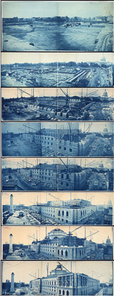
Construction of the Thomas Jefferson Building, from July 8, 1888 to May 15, 1894.
