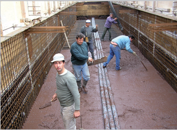
Concrete pouring top wall Dutch Floating breakwater elements
