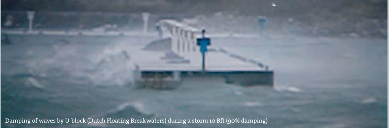
Turning U-Blocks (Dutch floating Breakwaters) in the water
