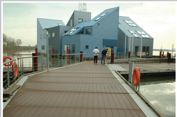
Fiber reinforced lightweight concrete elements, Amsterdam
