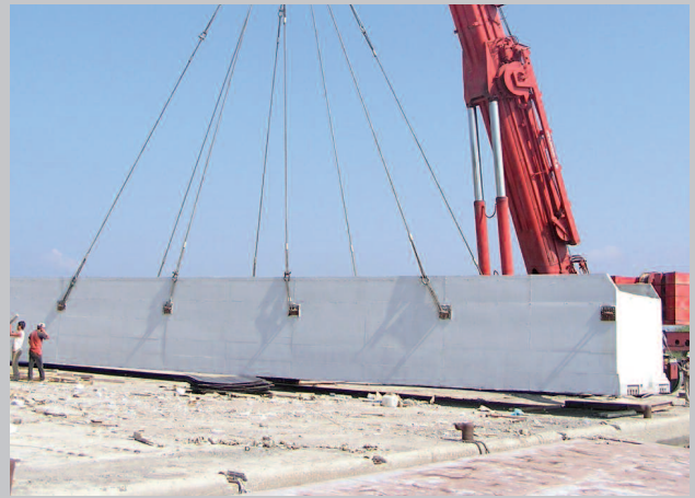
Standard U-Blocks (Dutch floating Breakwaters) 135 tons lifted by crane
