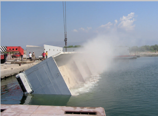
Turning U-Blocks (Dutch floating Breakwaters) in the water
