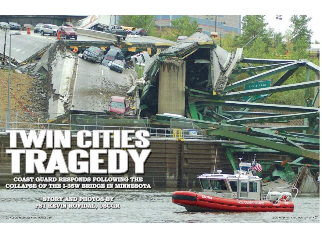
ust after 6 p.m. on Aug. 1, the I-35W bridge gave way and collapsed into the Mississippi River in Minneapolis, Minn. Resurfacing renovations were under way at the time of the accident, and there were several pieces of heavy construction equipment, building materials, and more than 100 vehicles on the bridge.
