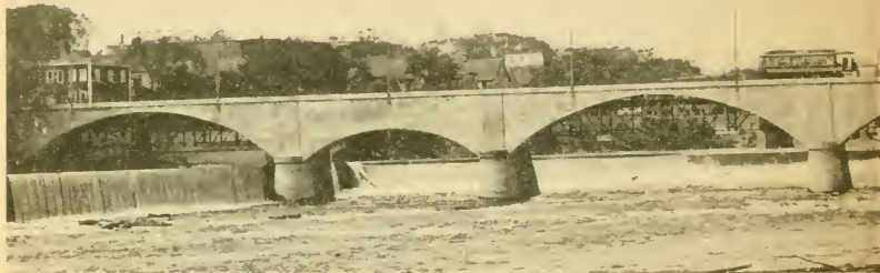
Trolley Bridge Into Waterville
