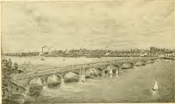
Crossing to the "East Side"
