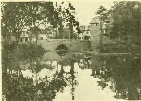
Milford Memorial Bridge
