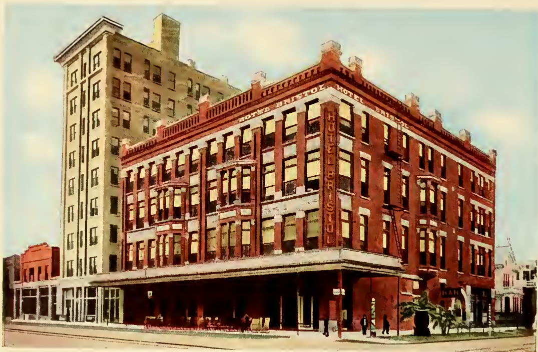
The Bristol Hotel and Annex Is One of the Well-Known Hostelries of the City.
