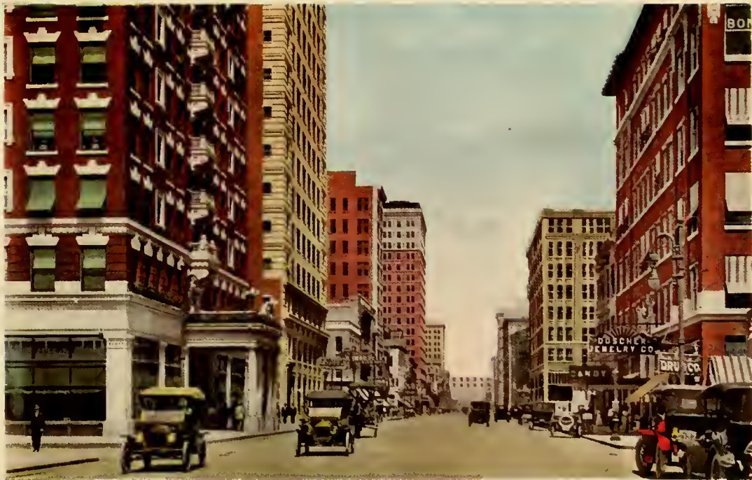
Main Street North From Walker Avenue. All the Buildings in This View Were Constructed Within the Last Three Years.
