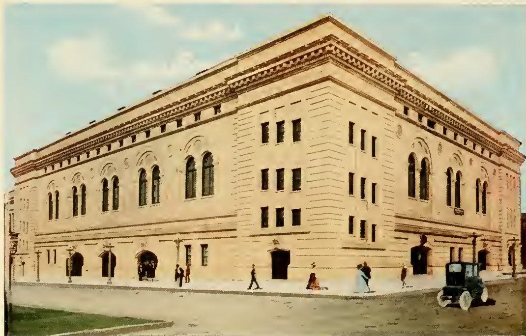
The City Auditorium Is the Largest Modern Convention Hall in the South. Seats 7,000 Persons and Cost $400,000.
