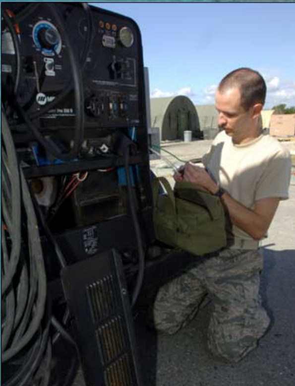
Senior Airman Nathan Ansell, an electrician with the 474 th Expeditionary Civil Engineering Squadron, strips wires to fit a new power source onto a generator, Feb. 26. – JTF Guantanamo photo by Army Spc. Carlynn M. Knaak
