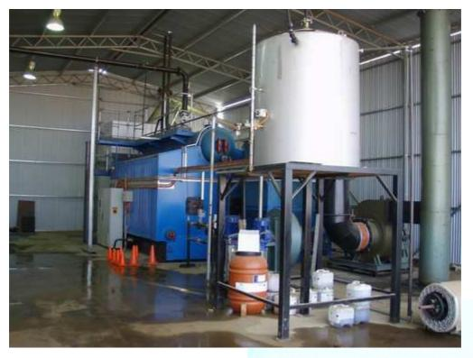
This is woodchip, sawdust, waste wood fuel, husks fired steam boiler :
