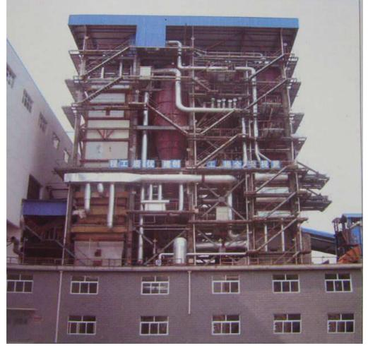
The boiler is circulation fluidized bed, include steam and hot water boiler, this is high pressure and steam, Larger industry and plant coal fired boiler.
