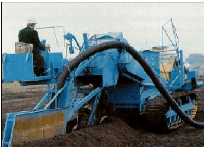
Installing drainage tile. Drainage tile is used extensively in central Illinois to remove excess water from farmland.
