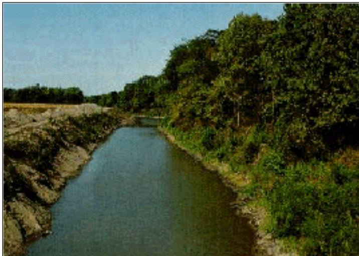
Balancing drainage and environmental considerations. This drainage ditch remains clear on one side. The trees that have been allowed to grow on the other side provide a habitat for wildlife.
