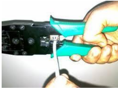
Figure 7: Crimping the cable
