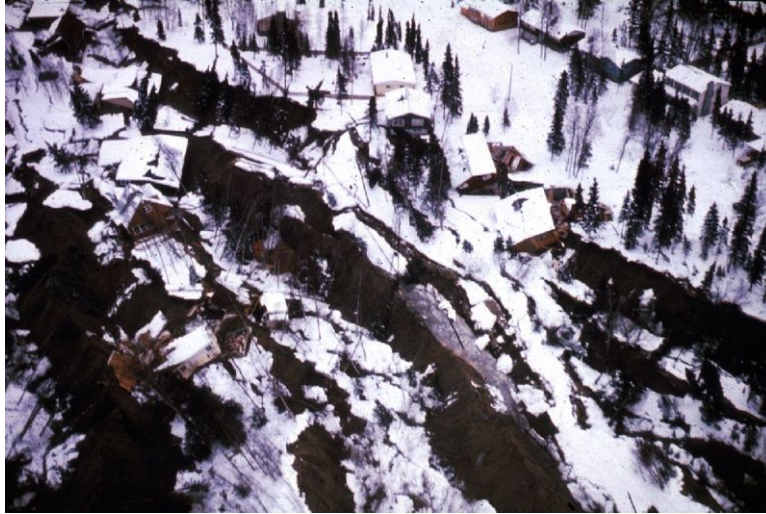
Figure 7.46: A landslide in a neighborhood in Anchorage Alaska after the 1964 Great Alaska earthquake. (29)
