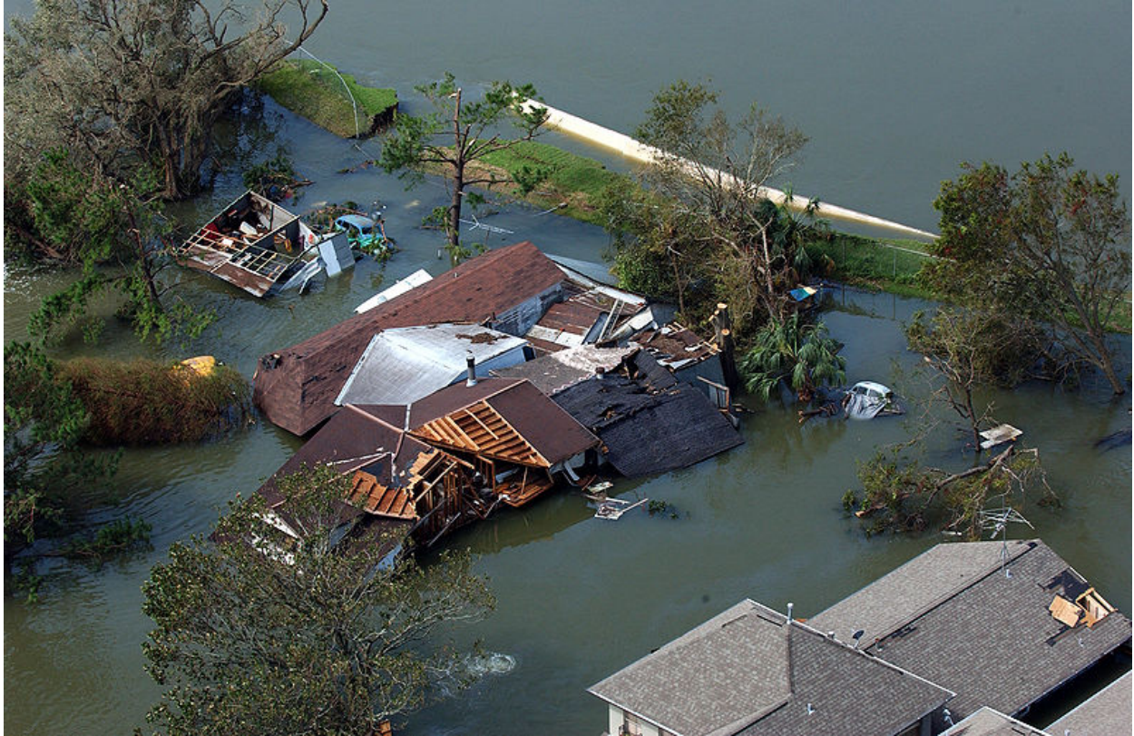
Figure 13.19: Levees that held back flood water were broken in many key areas around the city of New Orleans. (2)
