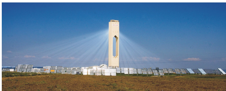
Figure 5.8: This solar power plant uses mirrors to focus sunlight on the tower in the center. The sunlight heats a liquid inside the tower to a very high temperature, producing energy to make electricity. (9)
