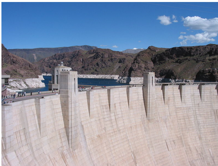
Figure 13.7: Hoover Dam on the Colorado River. (24)
