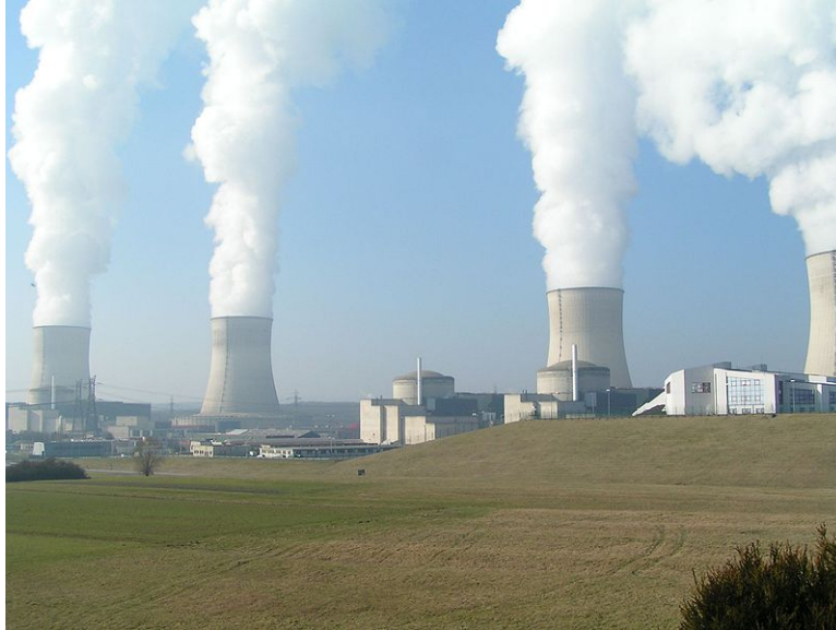
Figure 5.5: Nuclear power plants like this one provide France with almost 80% of its electricity. (6)
