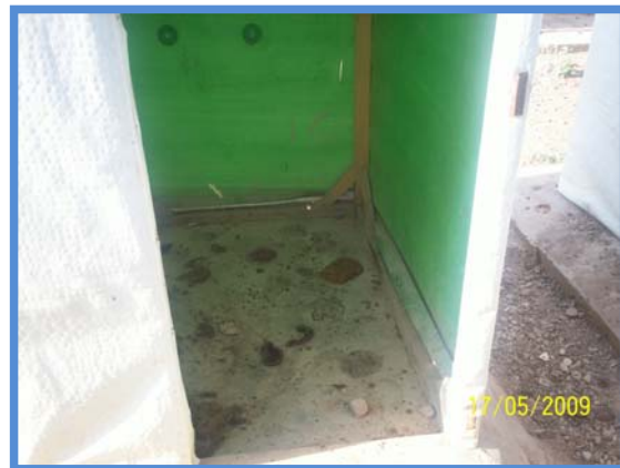
Figure 17. Wash rooms are being used as toilets in almost all camps
