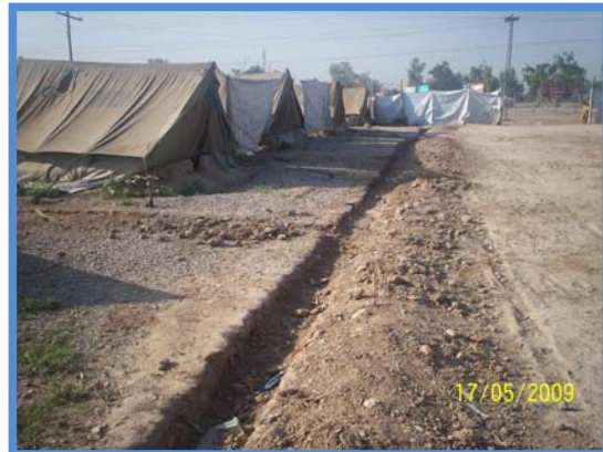
Figure 9. Waste and rain water collection ditches at Kacha Ghari Camp
