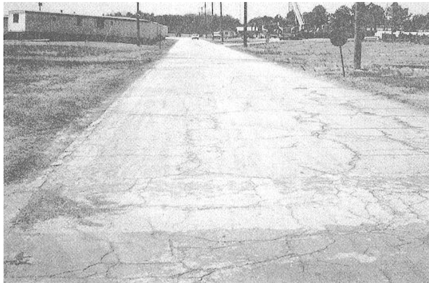
Figure 3-3. Block cracking.
