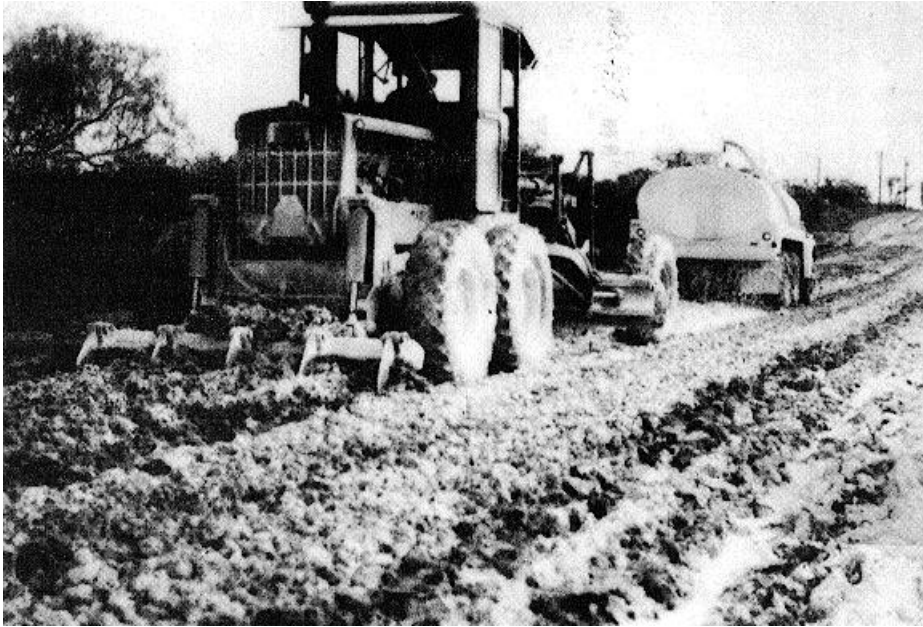
Figure 5-16. Spraying lime from a tank truck and immediately mixing treated soil.
