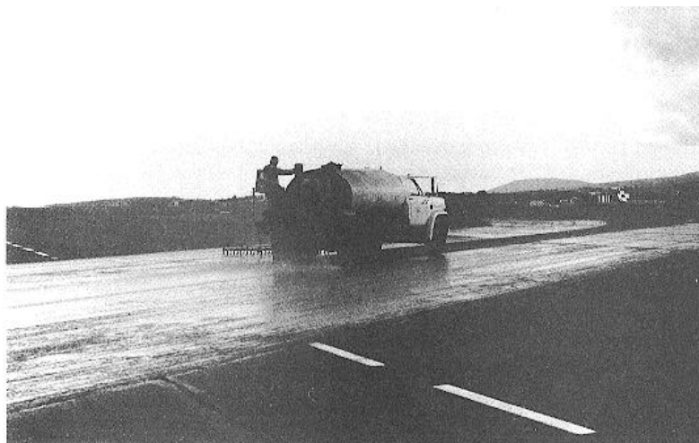
Figure 3-52. Applying rejuvenator
