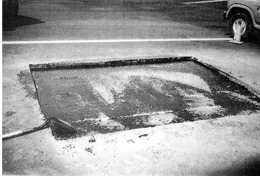
Figure 3-48. Hole to be patched with tack applied
