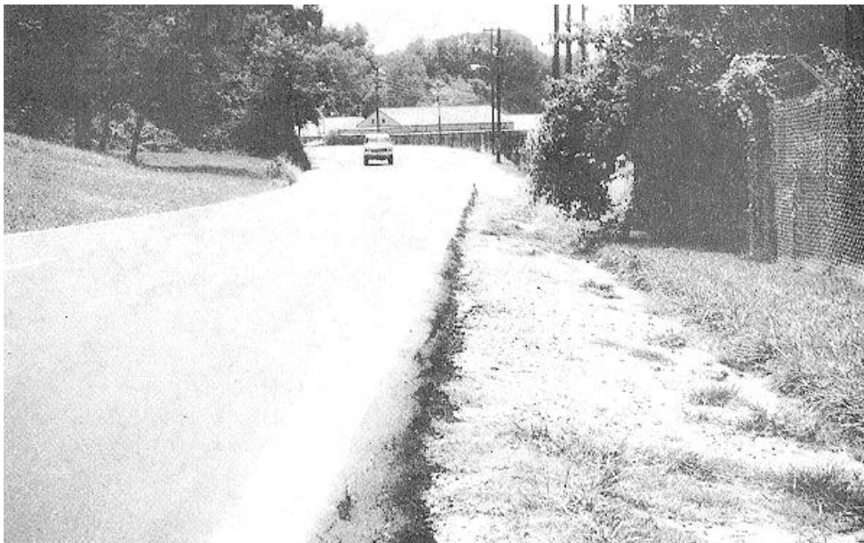
Figure 3-9. Lane/shoulder dropoff.
