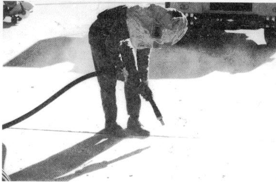
Figure 4-27. Blowing out dirt from joints.
