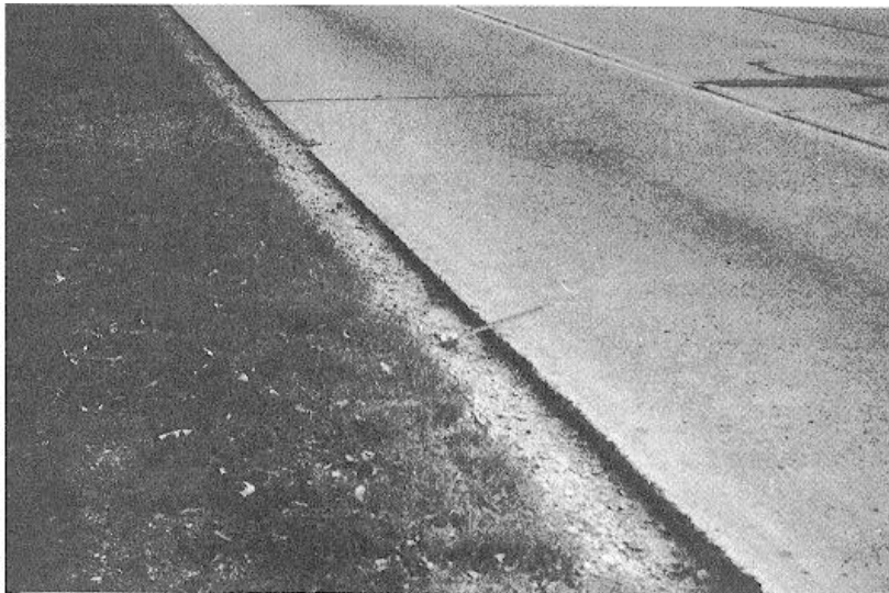
Figure 4-11. Lane/shoulder dropoff.
