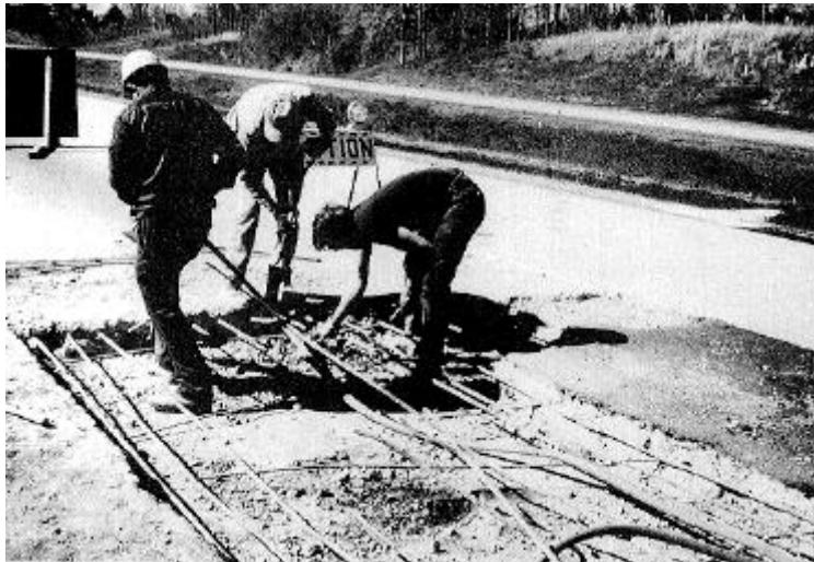
Figure 4-39. Placing reinforcement and dowels in area to be repaired.
