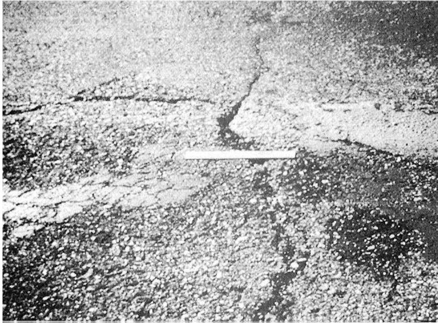
Figure 3-20. Weathering.
