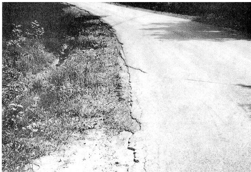
Figure 3-7. Edge cracking.
