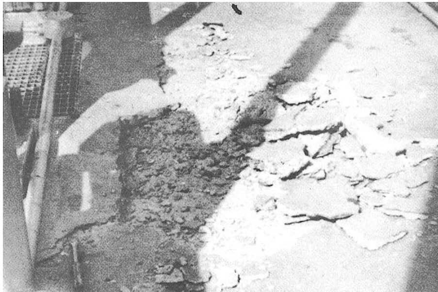
Figure 4-20. Scaling.
