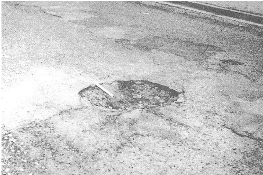
Figure 3-13. Potholes.
