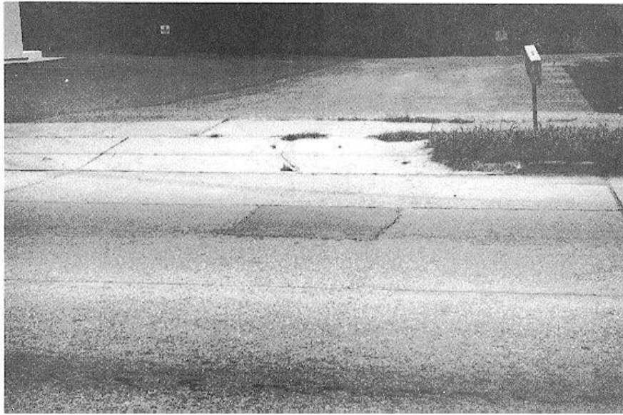
Figure 4-13. Utility cut patch.
