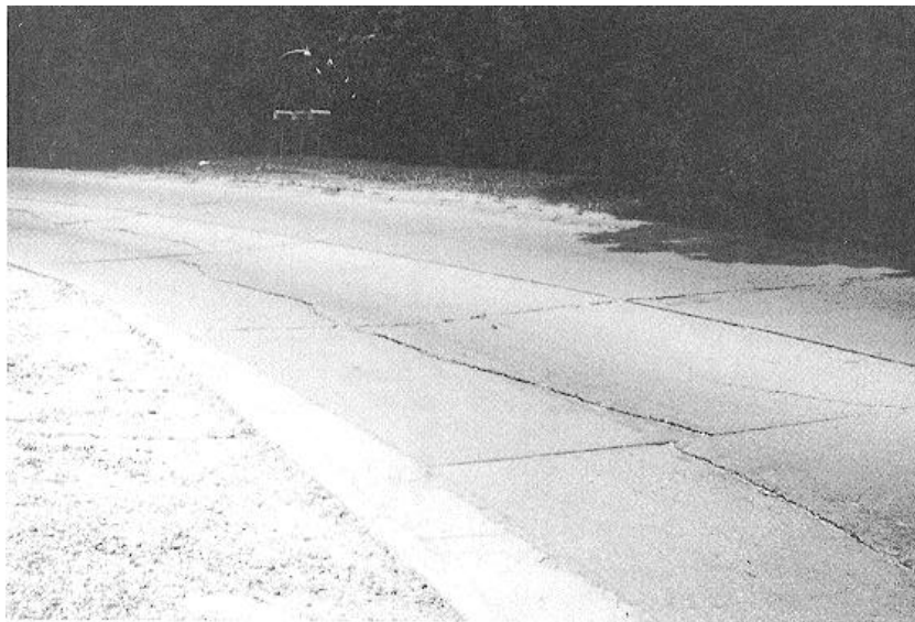
Figure 4-12. Liner cracking.
