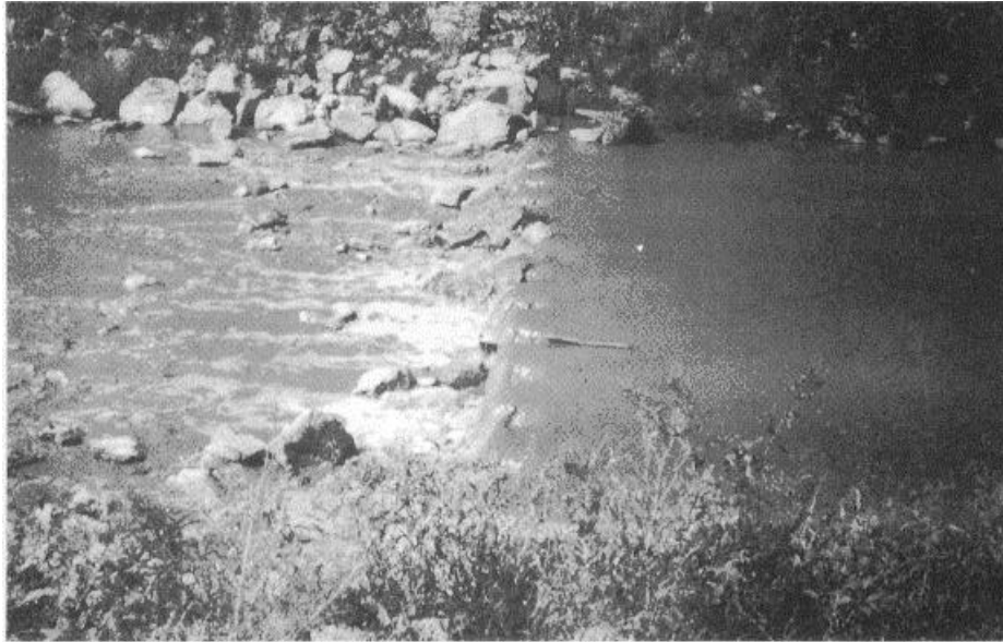
Figure 7-5. Ditch check.
