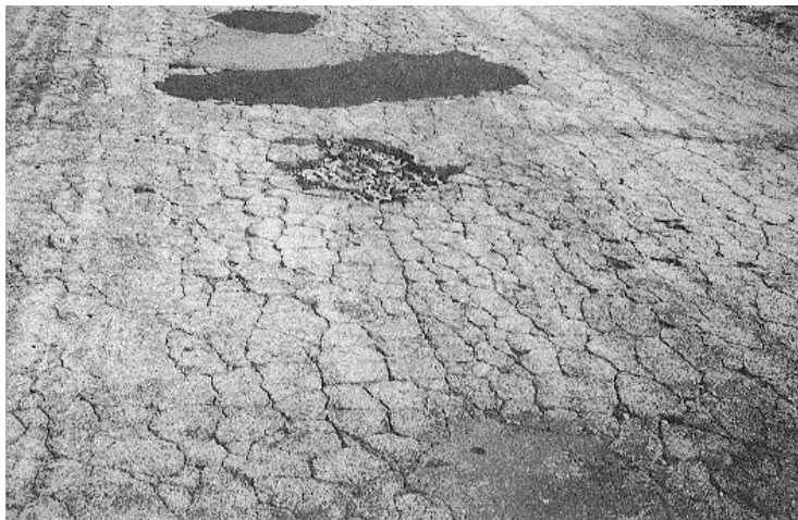
Figure 3-1. Alligator cracks.
