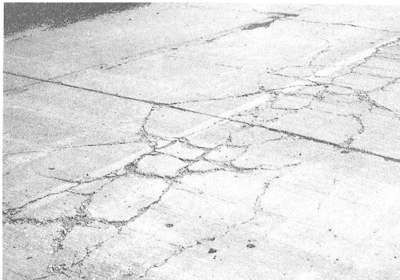
Figure 4-18. Punch out.
