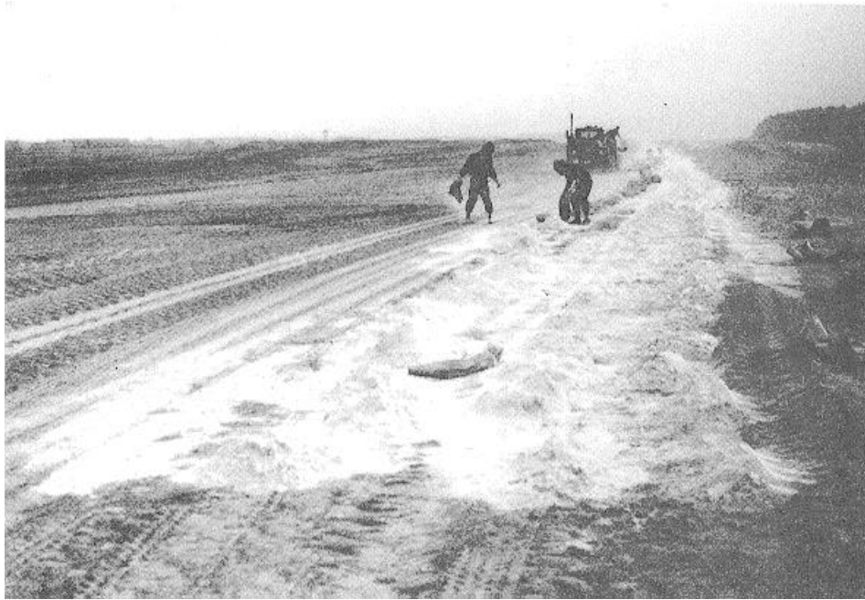
Figure 5-10. Hand spreading bags of cement.
