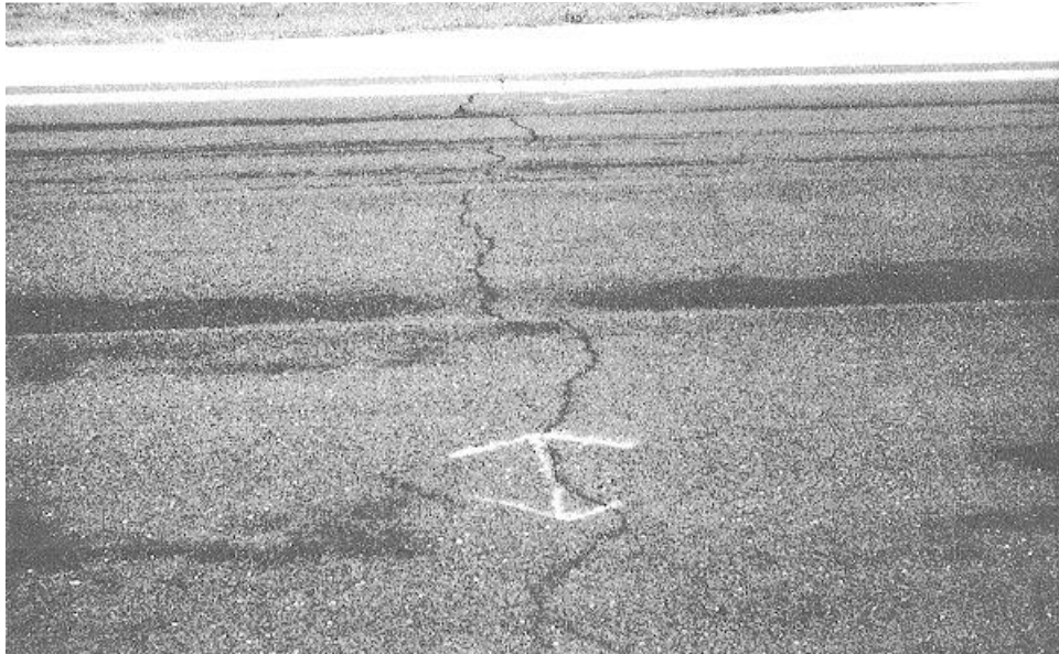
Figure 3-10. Transverse crack.
