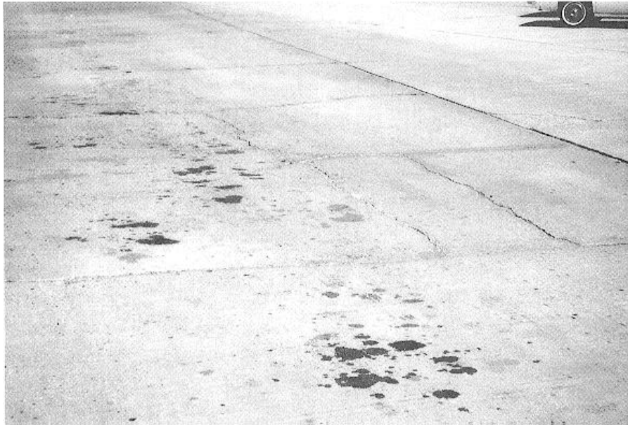
Figure 4-7. Divided slab.
