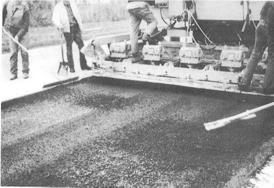
Figure 3-31. Scarified and bladed bituminous material being immediately respread and compacted.
