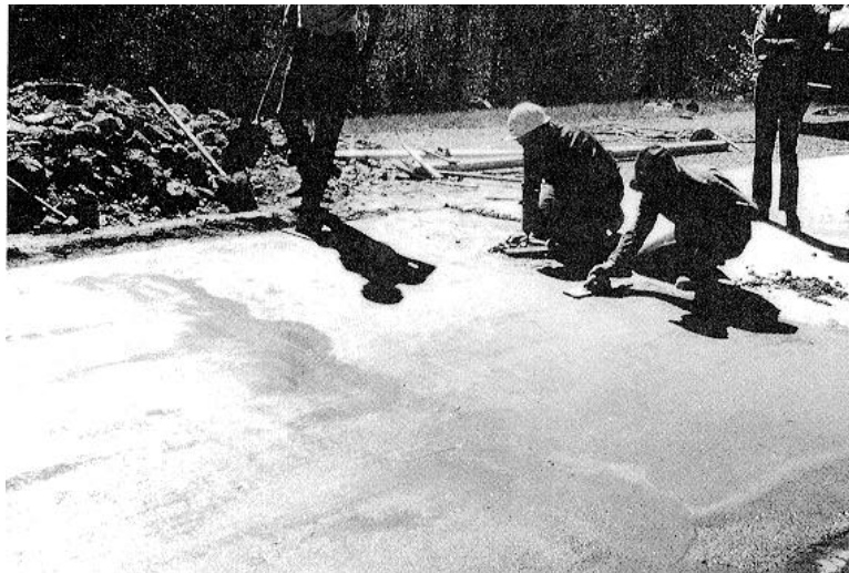
Figure 4-41. Finishing surface of concrete patch.-
