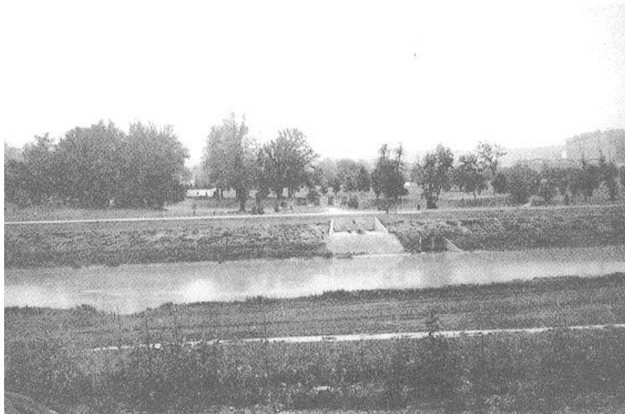
Figure 7-3. Concrete flume for discharging water into drainage channel.
