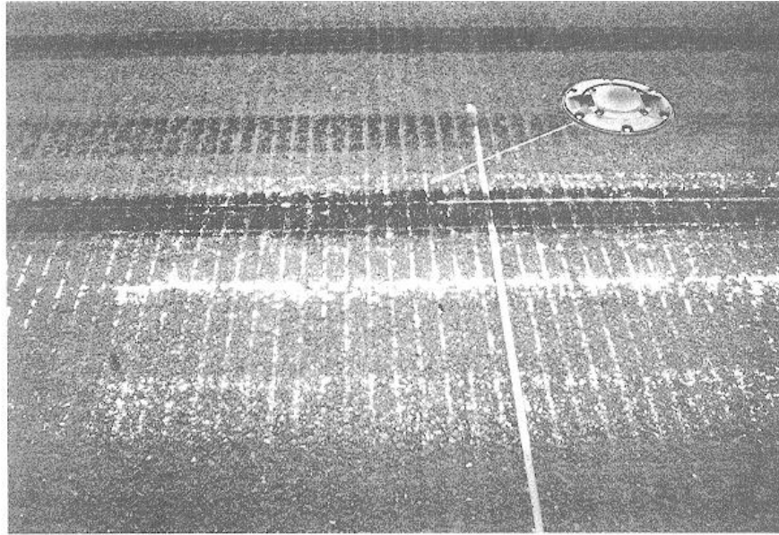
Figure 3-22. Grooved asphalt concrete pavement.
