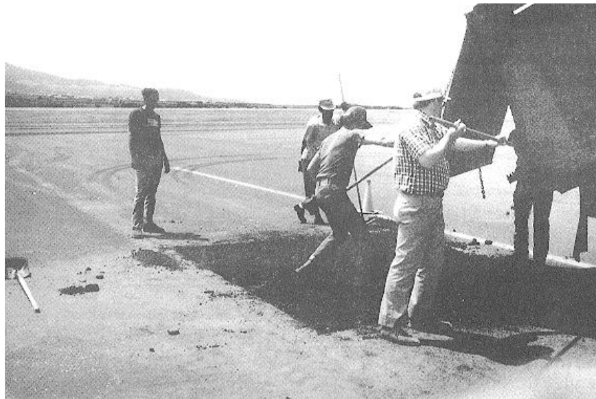
Figure 3-49. Placing asphalt mix in patch.
