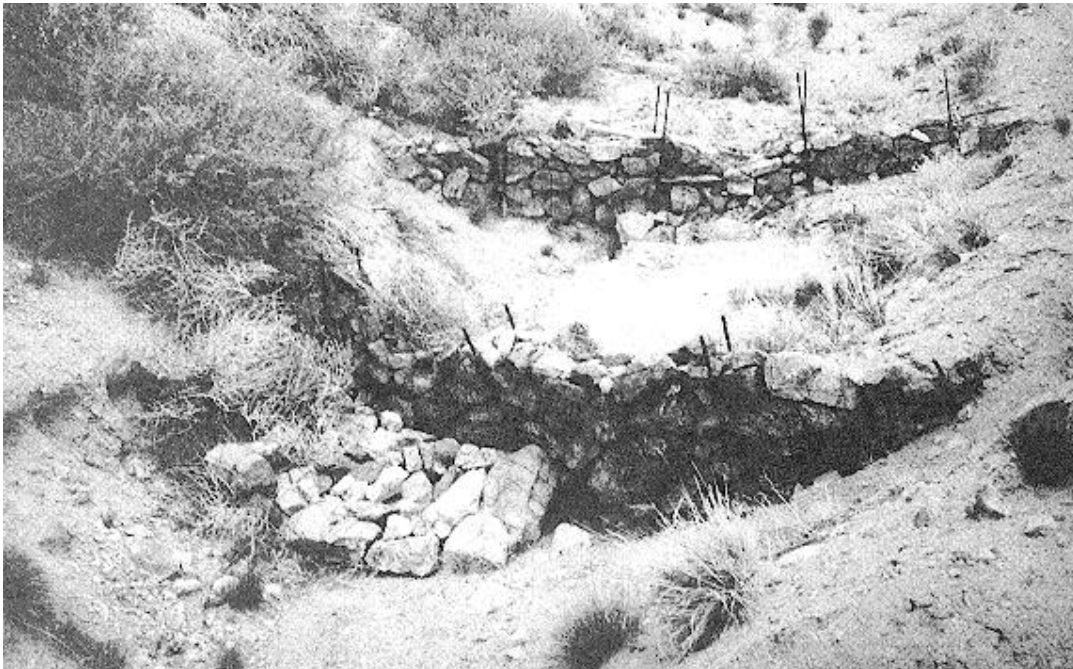
Figure 7-13. Rock fences for control of erosion.
