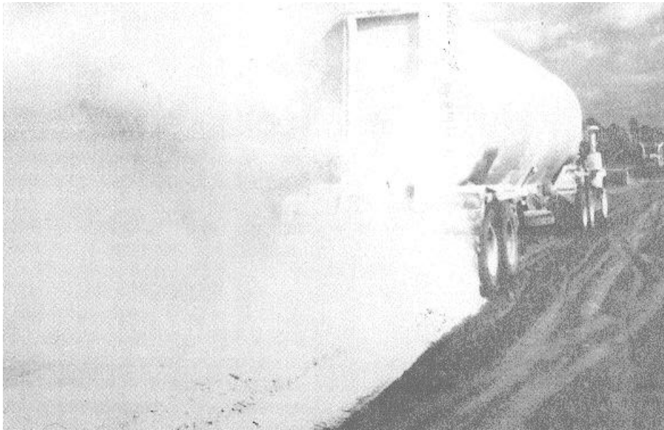
Figure 5-12. Spreading cement directly from bulk carrier.
