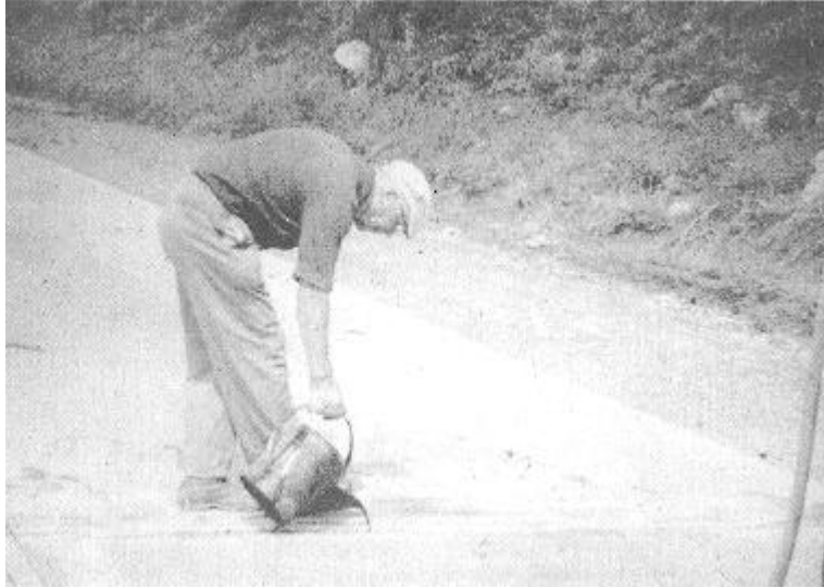
Figure 4-32. Applying crack sealer with a pouring pot.
