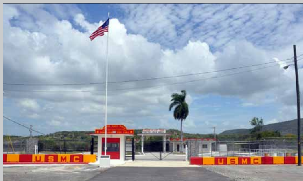
The North East gate after an approximately $70,000 renovation project including fresh paint, new concrete, and the removal of debris. The upgrade was facilitated by four Seabees attached to NAVFAC Southeast PWD and NMCB 23 and took more than 300 hours to complete.
